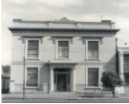
B0208 House Bank St South Melbourne
