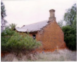
SW 02e - brick building adjacent to main homestead building.
