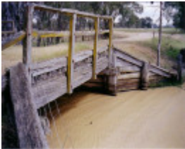
TU 01 - Timber Bridge, old Tulkara Navarre Road over Heifer Station Creek tributary, TULKARA
