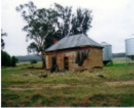
WI 01 - Derelict Mud Brick House, Barkly Gap Road, WINJALLOCK
