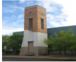
Massey Ferguson Complex_Sunshine_Clock Tower _Sept 2007
