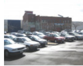
Massey Ferguson Complex_Sunshine_Stores Building_Sept 2007_01
