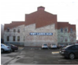
Massey Ferguson Complex_Sunshine_Stores Building_Sept 2007_02
