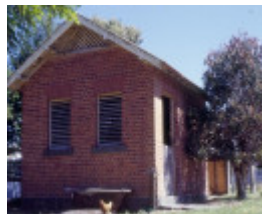
h00533 former police residence and lock up heales street talbot stables she project 2003
