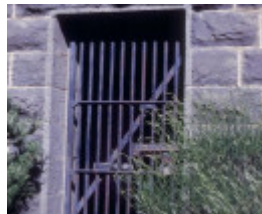
h00533 former police residence and lock up heales street talbot lock up gate she project 2003
