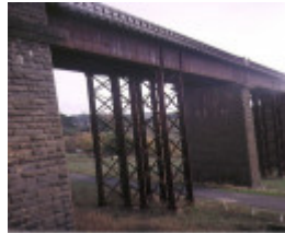
1 railway viaduct heales street taradale side elevation apr1995
