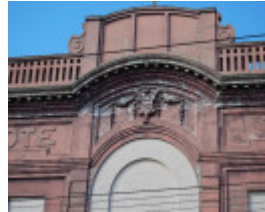
11447 Northcote Cinema 212 220 High Street Facade Detail 1 31
