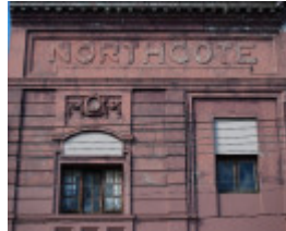
11447 Northcote Cinema 212 220 High Street Facade Detail 2 31
