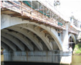
CHURCH STREET BRIDGE SOHE 2008
