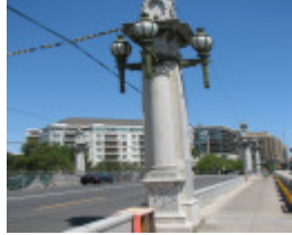
CHURCH STREET BRIDGE SOHE 2008
