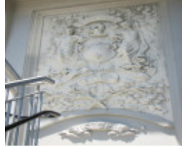
CHURCH STREET BRIDGE SOHE 2008
