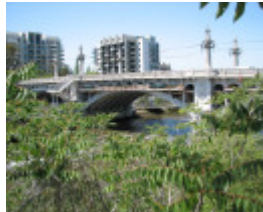
CHURCH STREET BRIDGE SOHE 2008
