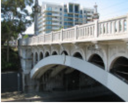
CHURCH STREET BRIDGE SOHE 2008
