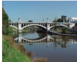
1 church street bridge from se bank mar01
