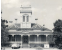
B1680 House 10 Queens Rd Melbourne
