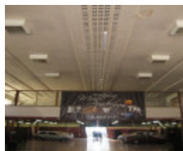
11488 Royal Melbourne Regiment Drill Hall Drill Hal Ceiling 11 Sept 2006 mz
