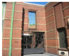
11488 Royal Melbourne Regiment Drill Hall Exterior Detail 02 11 Sept 2006 mz
