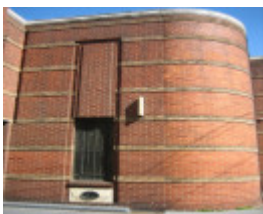
11488 Royal Melbourne Regiment Drill Hall Exterior Detail 01 11 Sept 2006 mz
