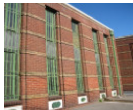
11488 Royal Melbourne Regiment Drill Hall Exterior Window Detail 11 Sept 2006 mz
