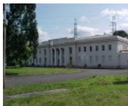
1 former yallourn power station administrative building
