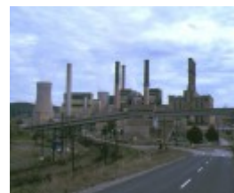
1 yallourn a b c d & e power stations latrobe valley yallourn property view
