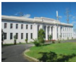
FORMER YALLOURN POWER STATION ADMINISTRATIVE BUILDING SOHE 2008
