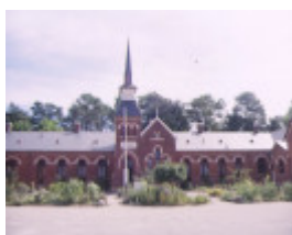
beechworth primary school no 1560 junction road beechworth front elevation mar1998
