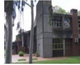
Example of 1970s college building.jpg
