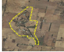
Aerial of Glenormiston Extent.jpg
