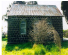
1 lutheran church gardenia road thomastown rear view
