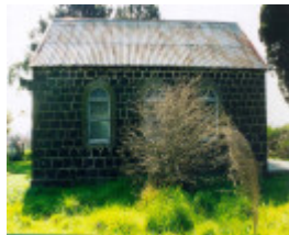
1 lutheran church gardenia road thomastown rear view
