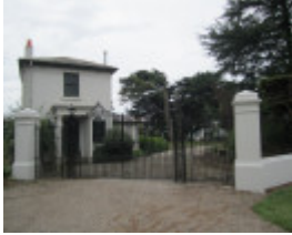
Front entrance showing Gatehouse
