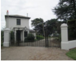
Front entrance showing Gatehouse
