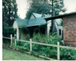
Dunbar Cottage and Dairy
