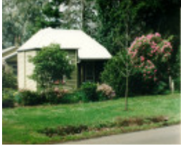
Dunbar Cottage and Dairy
