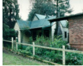
Dunbar Cottage and Dairy
