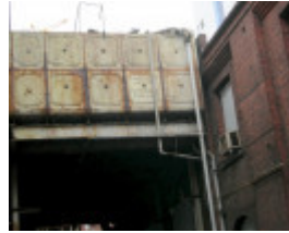
OVERHEAD WATER TANK SOHE 2008
