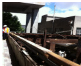
remedial works commence Nov 2011
