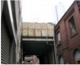
OVERHEAD WATER TANK SOHE 2008
