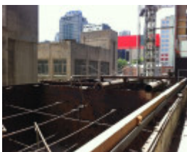
Internal tie rods
