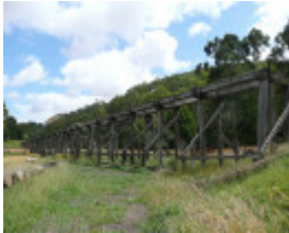
RAIL BRIDGE SOHE 2008
