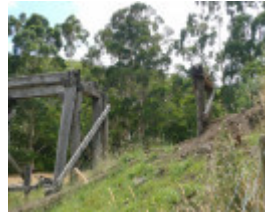
RAIL BRIDGE SOHE 2008
