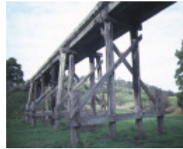
rail bridge curdies river timboon trestle detail jun1984
