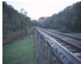
rail bridge curdies river timboon rail tracks jun1984
