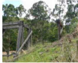
RAIL BRIDGE SOHE 2008
