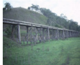
1 rail bridge curdies river timboon side view jun1984
