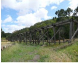
RAIL BRIDGE SOHE 2008
