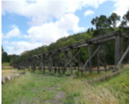
RAIL BRIDGE SOHE 2008
