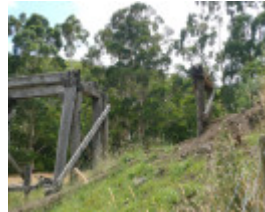
RAIL BRIDGE SOHE 2008
