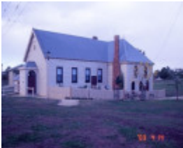
h00544 mechanics institute free library king and cowan street toongabbie south west view she project 2003
