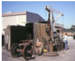
Former Railway Workshops Champion Road Newport Hydraulic Crane
