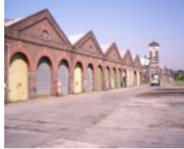
1 former railway workshops champion road newport east block of workshops feb1994
