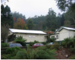
side of building
