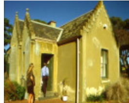
1 overnewton gatehouse h1947 march 2001
