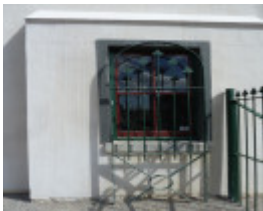
H1947 OVERNEWTON GATEHOUSE LHA 2015 2.JPG
