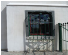
H1947 OVERNEWTON GATEHOUSE LHA 2015 2.JPG
