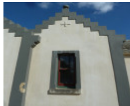
H1947 OVERNEWTON GATEHOUSE LHA 2015 4.JPG
