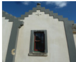
H1947 OVERNEWTON GATEHOUSE LHA 2015 4.JPG
