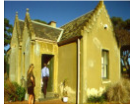
1 overnewton gatehouse h1947 march 2001
