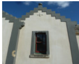
H1947 OVERNEWTON GATEHOUSE LHA 2015 4.JPG
