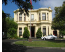
Main facade to Irving Road
