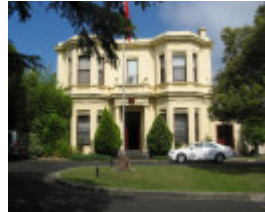
Main facade to Irving Road
