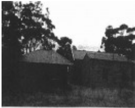
Former School & Mechanics Institute
