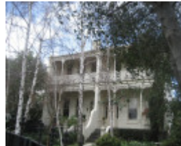
Victorian terrace, 52-54 Chatsworth Road.
