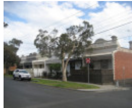
Victorian terrace, 39-49 Chatsworth Road.
