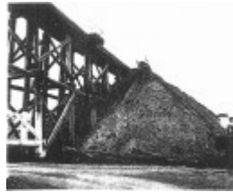
Melbourne-Ballarat Railway Bridge
