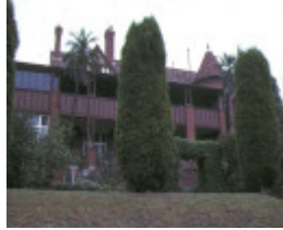
1 edzell st georges road toorak front view may1988
