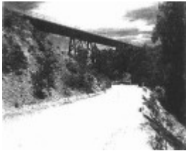
Railway Viaduct, Bridge and Embankment
