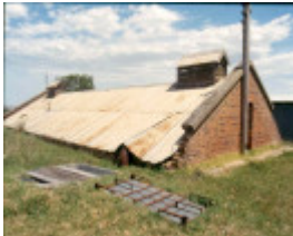
h02040 bairnsdale pumping station 1888 brick tank
