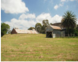
BAIRNSDALE PUMPING STATION SOHE 2008
