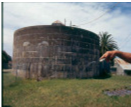
h02040 bairnsdale pumping station monier 1906 tank
