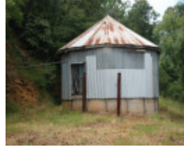
BAIRNSDALE PUMPING STATION SOHE 2008
