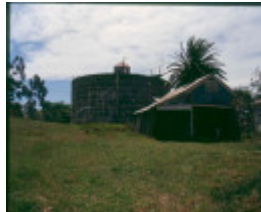
h02040 bairnsdale pumping station 2002
