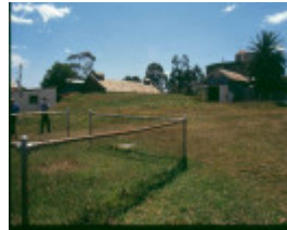
h02040 bairnsdale pumping station 2 2002
