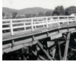
B4134 Timber Trestle Bridge
