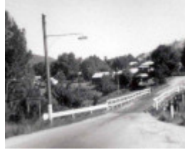
B4134 Timber Trestle Bridge
