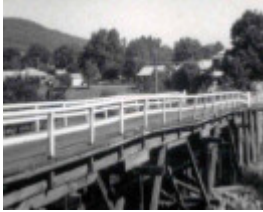
B4134 Timber Trestle Bridge
