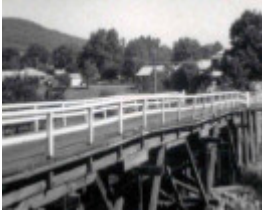
B4134 Timber Trestle Bridge
