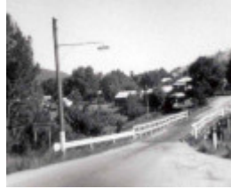
B4134 Timber Trestle Bridge
