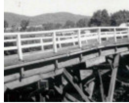
B4134 Timber Trestle Bridge
