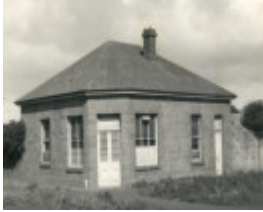
B1477 Cottage cnr Palmer & Otway Sts Portland
