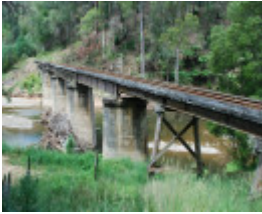
RAIL BRIDGE SOHE 2008
