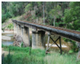
RAIL BRIDGE SOHE 2008
