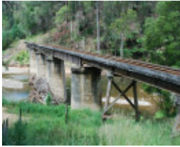
RAIL BRIDGE SOHE 2008
