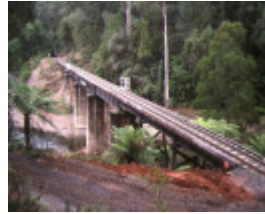
1 rail bridge thomson river walhalla end view apr1995
