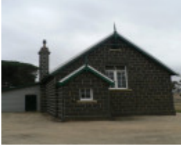
Former State School, now Public Hall, Murgheboluc
