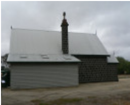
West elevation, Former State School, Murgheboluc
