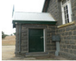
Entrance Porch, Former State School, Murgheboluc
