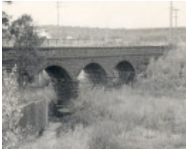
B0942 Bluestone Bridge
