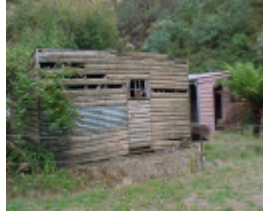
Walhalla Post Office Exterior Outbuildings March 2003
