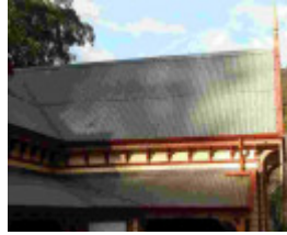
Before Photograph - Reference F3834 2014
