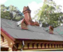
Before Photograph - Reference F3834 2014
