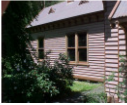
Walhalla Post Office Exterior Side March 2003
