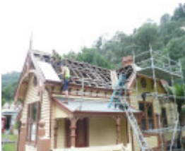
During Photograph - Reference F3834 2015
