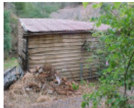
H00583 walhalla po exterior outbuilding mar 2003
