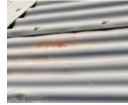
Before Photograph - Reference F3834 2014
