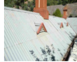
Before Photograph - Reference F3834 2014
