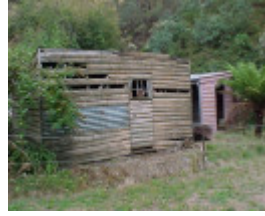
Walhalla Post Office Exterior Outbuildings March 2003
