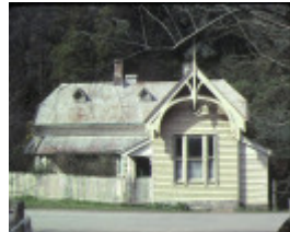
H00583 former walhalla post office walhalla front view sep1982
