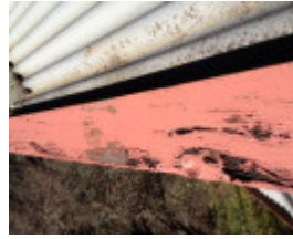
Before Photograph - Reference F3834 2014
