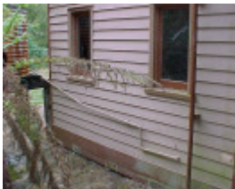
H00583 walhalla po exterior openings mar 2003
