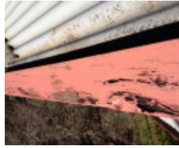
Before Photograph - Reference F3834 2014
