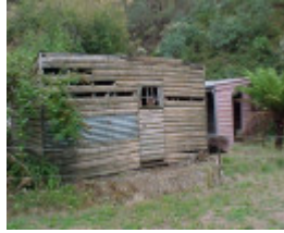
Walhalla Post Office Exterior Outbuildings March 2003
