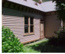
Walhalla Post Office Exterior Side March 2003
