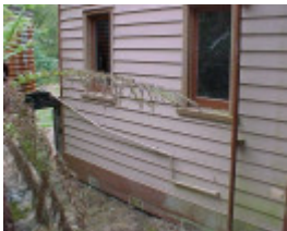
H00583 walhalla po exterior openings mar 2003
