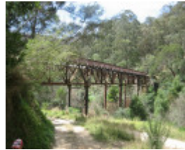
Bruntons Bridge Thompson River, 2006
