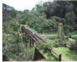
1 bruntons bridge thomson river narracan front view 1983
