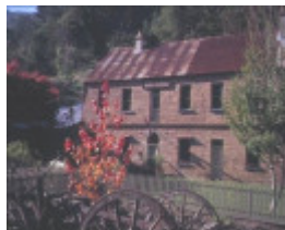
h00326 Windsor house right hand branch walhalla front view she project 2003
