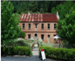
WINDSOR HOUSE SOHE 2008
