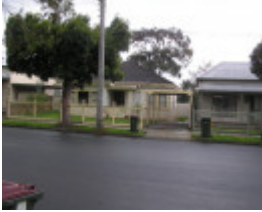
14 Waratah Street, Geelong West
