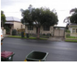
16 Waratah Street, Geelong West
