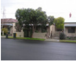
18 Waratah Street, Geelong West
