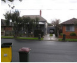
30 Waratah Street, Geelong West
