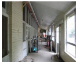
Recreation wing corridor
