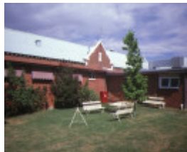
ovens & murray hospital for the aged warners road beechworth side elevation dec1984
