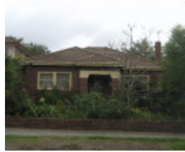
Interwar villa at 15 Allaville Avenue
