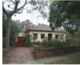
Interwar villa at 10 Allaville Avenue
