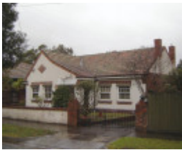
Interwar villa at 6 Allaville Avenue
