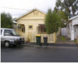
69 Waratah Street, Geelong West
