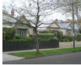
Edwardian timber villas on the west side of Warley Road
