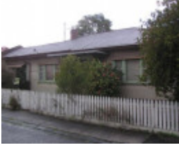
1 Plymouth Street, Geelong West
