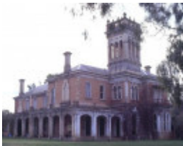
h00359 1 bontharambo homestead boorhaman road wangeratta south view she project 2003
