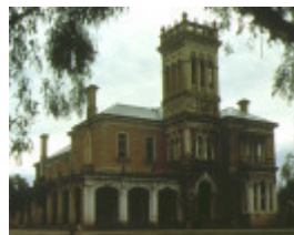
h00359 bontharambo homestead off boorhaman rd wangeratta front view homestead jun1978
