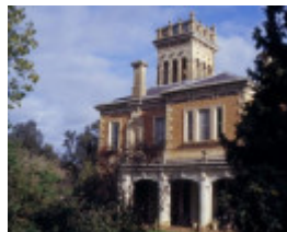
bontharambo homestead boorhaman road wangeratta view from garden she project 2003
