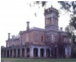
h00359 1 bontharambo homestead boorhaman road wangaratta south view she project 2003
