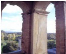
bontharambo homestead boorhaman road wangaratta view from tower she project 2003
