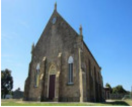
HO21 Uniting Church Old Western Highway Myrniong
