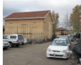
MMTB substation_Thornbury_14 May 2009_mz
