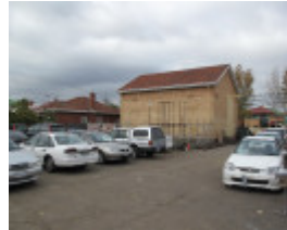
MMTB substation_Thornbury_14 May 2009_mz
